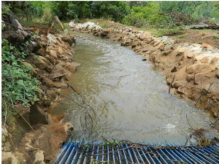
Canal end with screening grid to remove foreign objects
