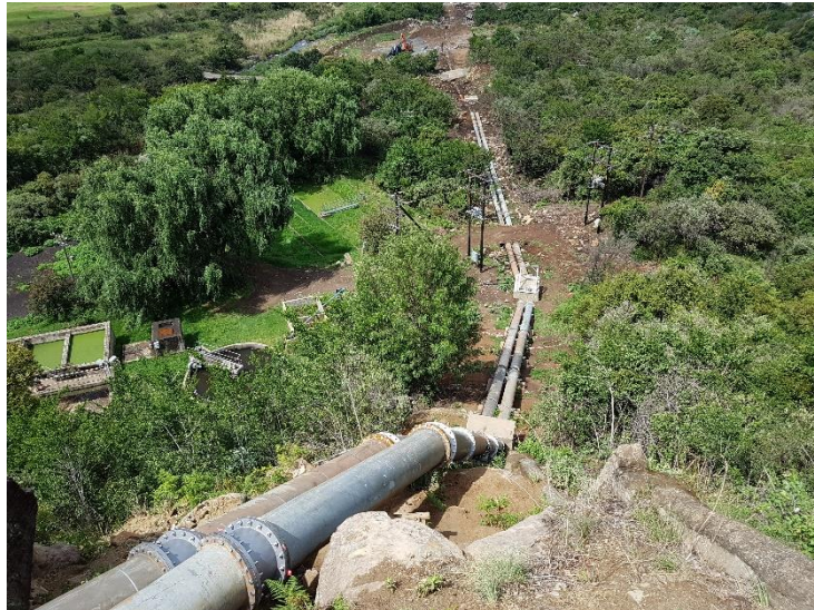
Penstock during construction
