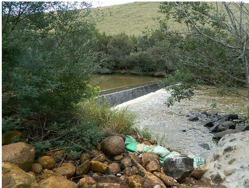
Weir in the Mooi River stretching 30m in total across the river.
